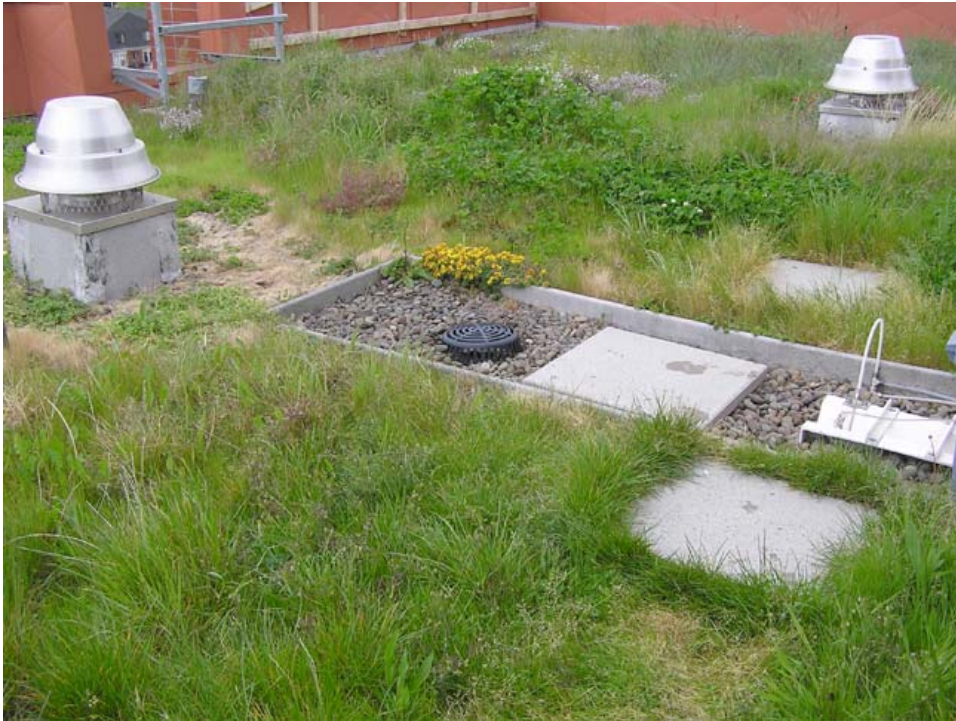
Hamilton West Apartments Green Roof, Portland Oregon
